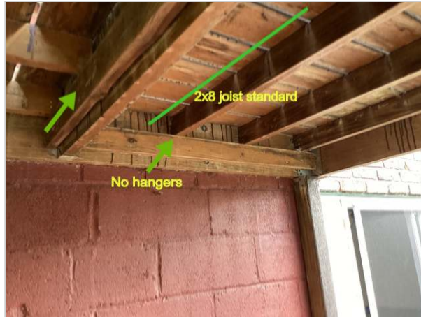
No joist hangers and 2 x4 joist
